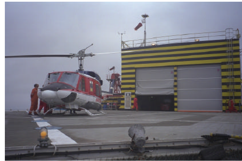
Offshore-door used as helicopter hangar-doors in the Northsea offshore doors are designed for windload at least 3000N/m 2
