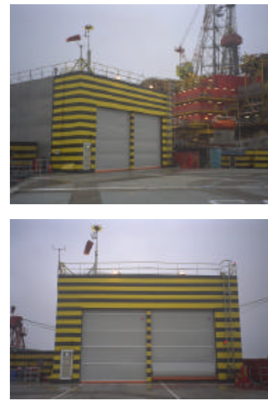
Offshore-door used as helicopter hangar-doors in the Northsea offshore doors are designed for windload at least 3000N/m 2
